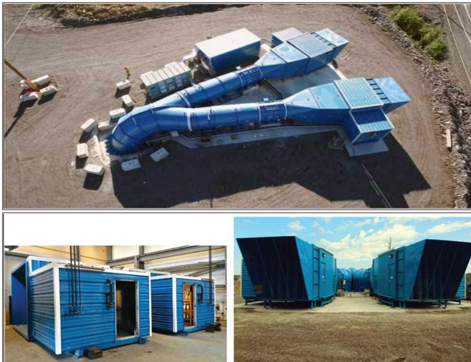
Figure 18-1: Typical Heating and Ventilation System for an Underground Portal
