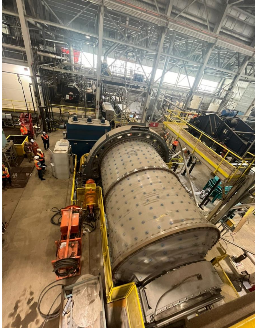
First ore grinding in early April
