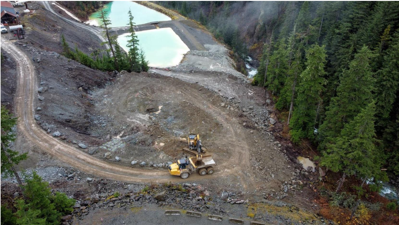
Figure 4 – Clarifier foundation preparation
