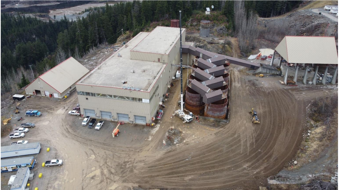
Figure 1 – Mill building area graded
