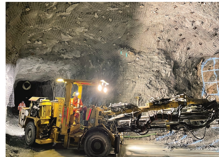
Underground development at the Big Missouri deposit
