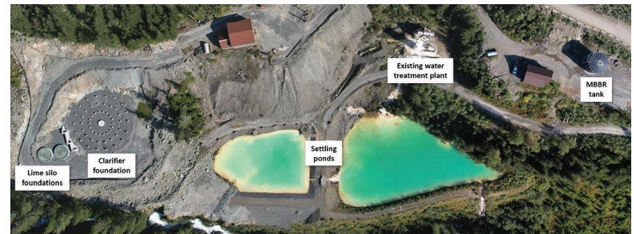
TOP: Dago Pit water collection facility at Big Missouri
