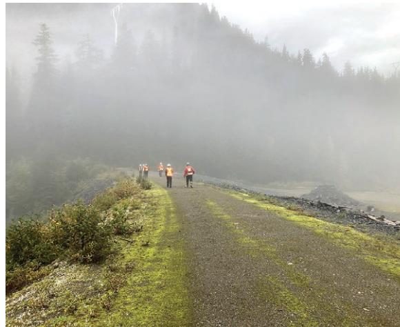
Routine tailings facility inspection on the south dam
