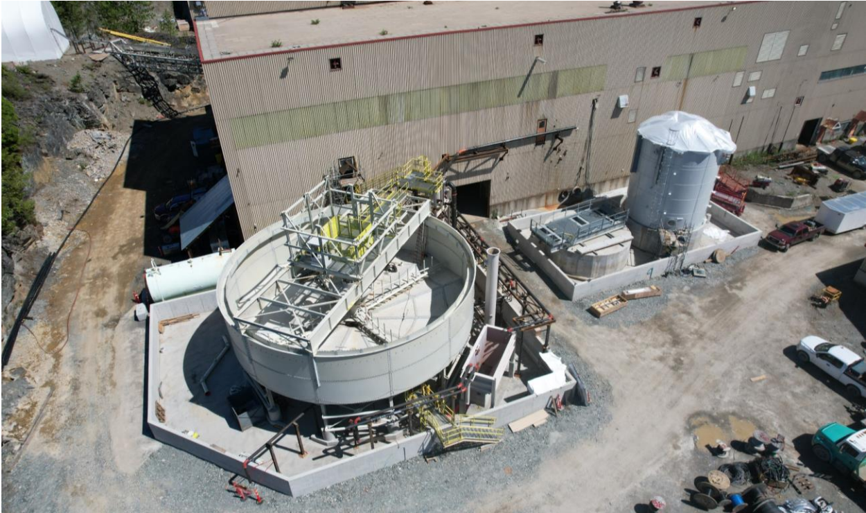
Figure 5 – Tailings thickener and CN destruction tank
