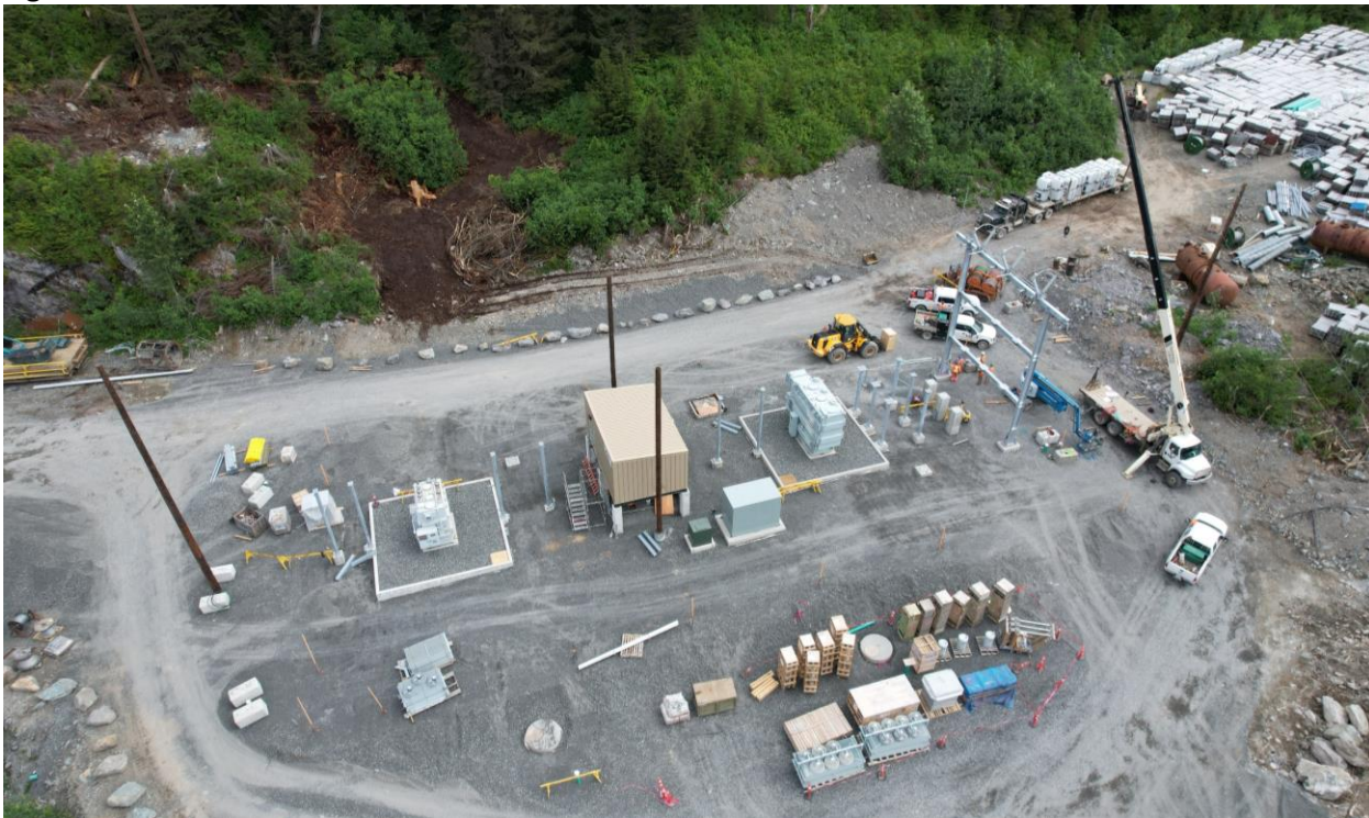
Figure 1 – New electrical substation construction
