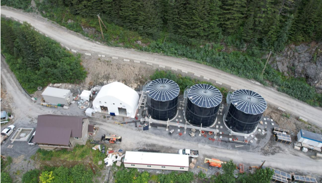
Figure 4 – New WTP MBBR tanks and electrical building
