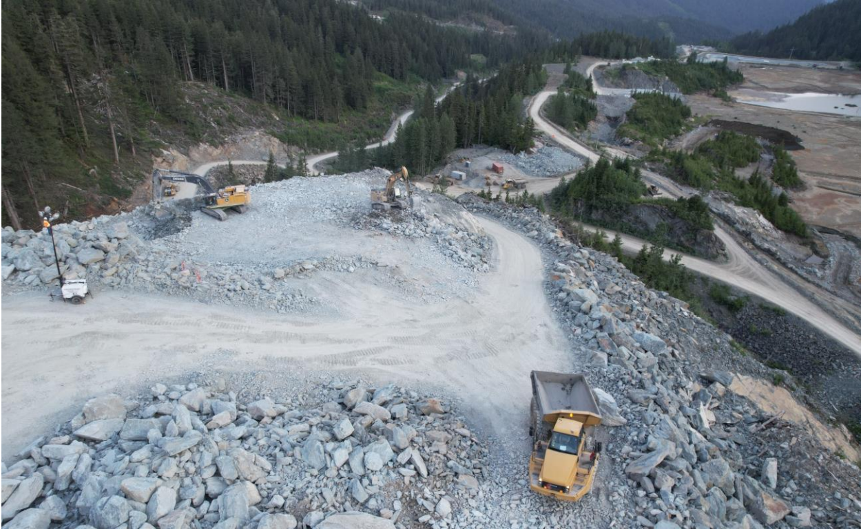
Figure 7 – CCDC excavation looking south
