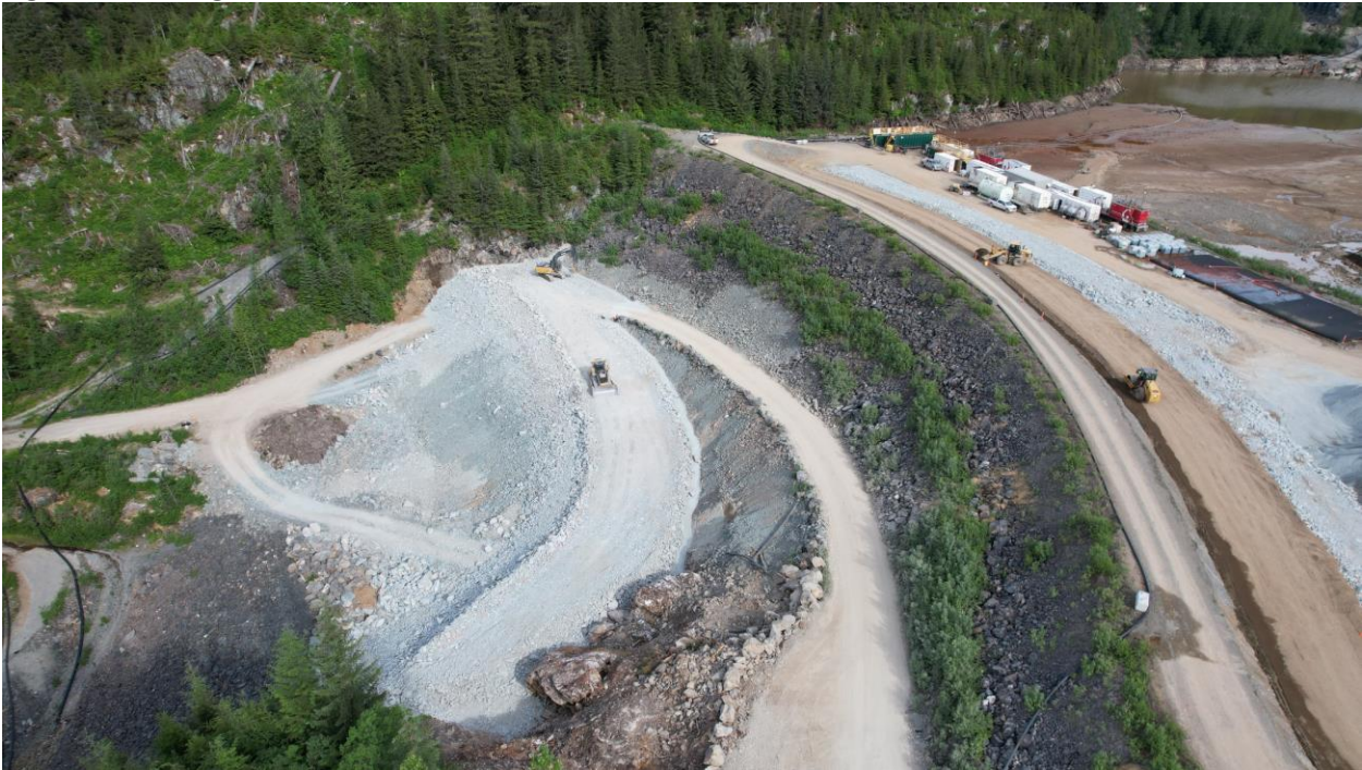
Figure 8 – Tailings south dam earthworks
