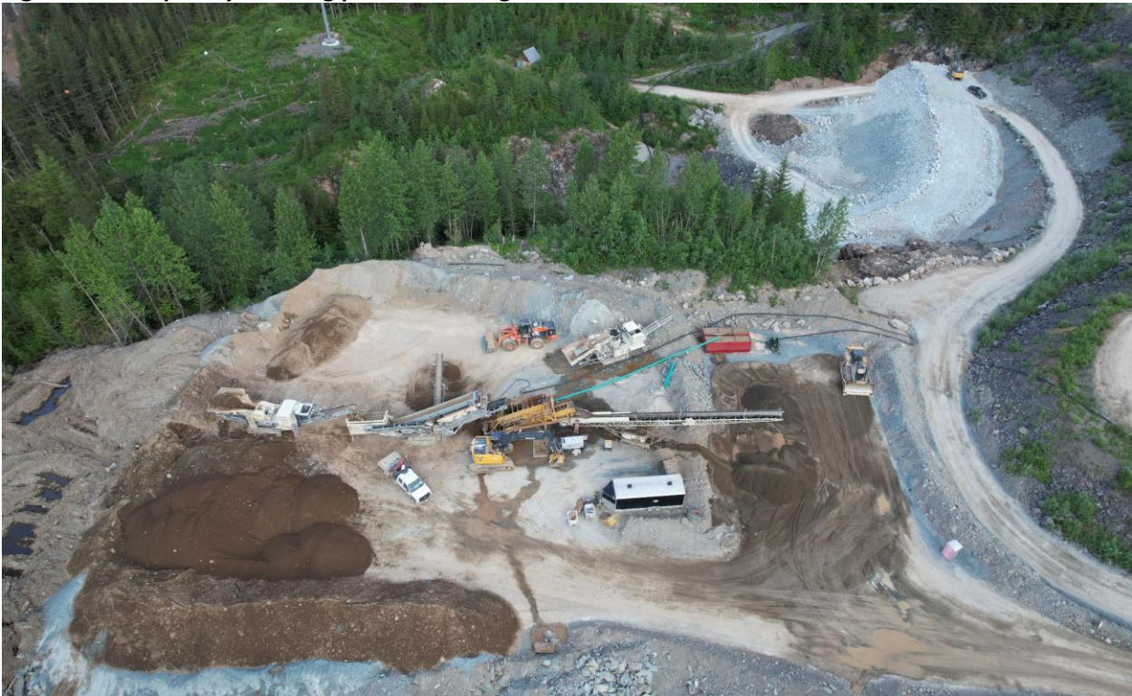
Figure 9 – Temporary crushing plant for tailings earthworks
