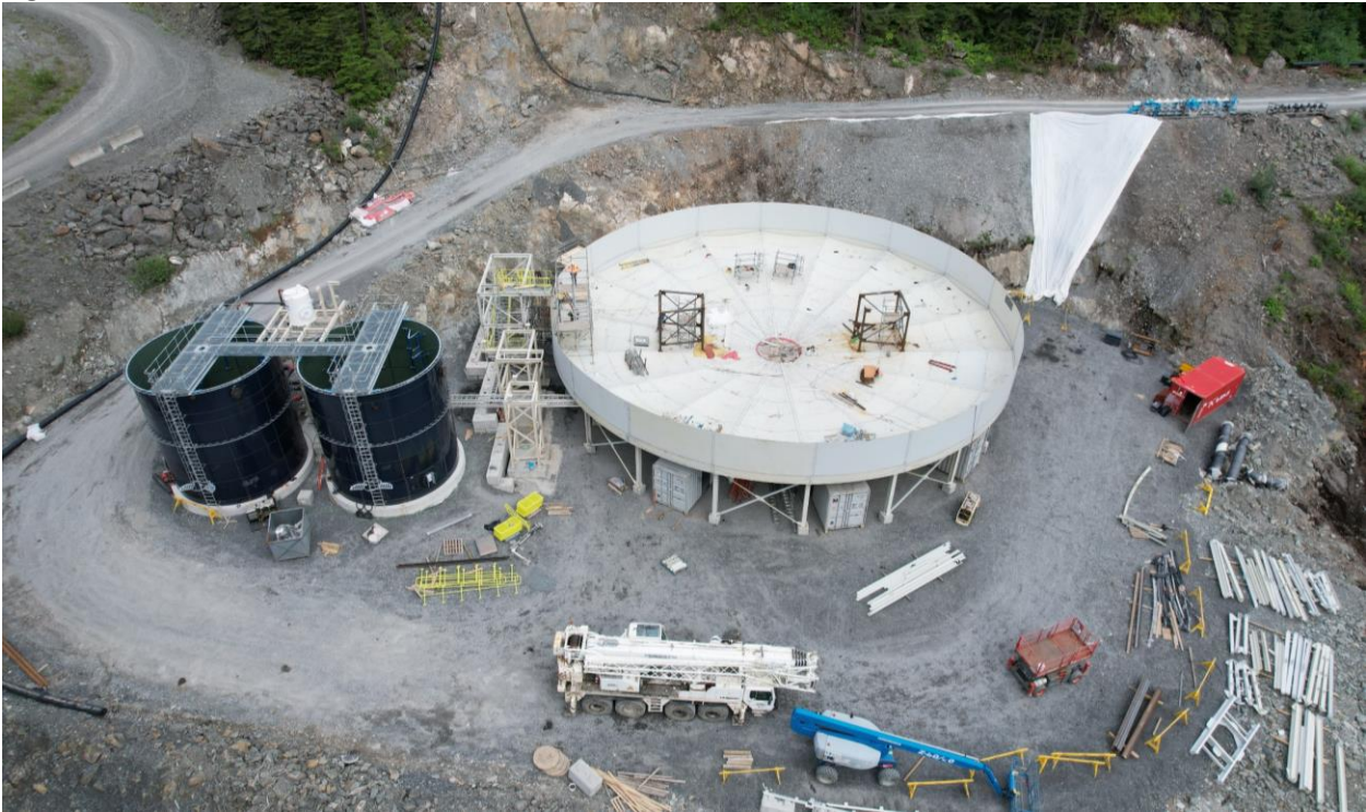
Figure 3 – New WTP clarifier construction
