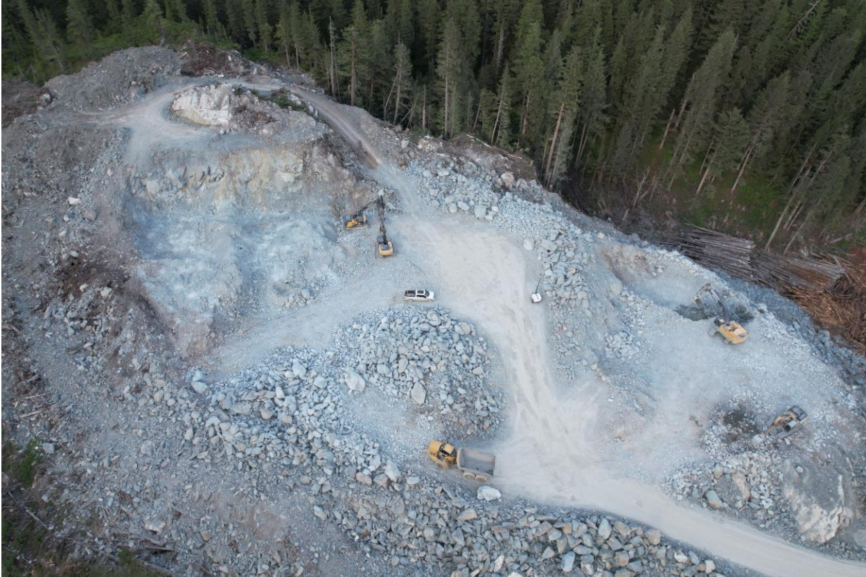
Figure 6 – CCDC excavation overview
