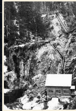
1956 – A fire burns down the Premier mill
