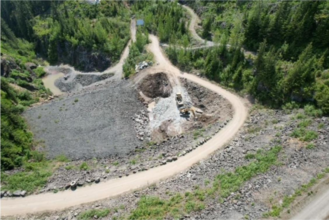
Figure 6 – Cascade Creek diversion channel excavation
