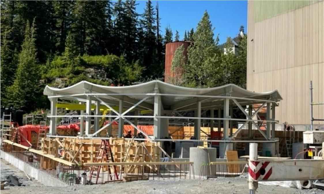
**Figure 3 – Tailings thickener and cyanide destruction tank erection outside mill building**
