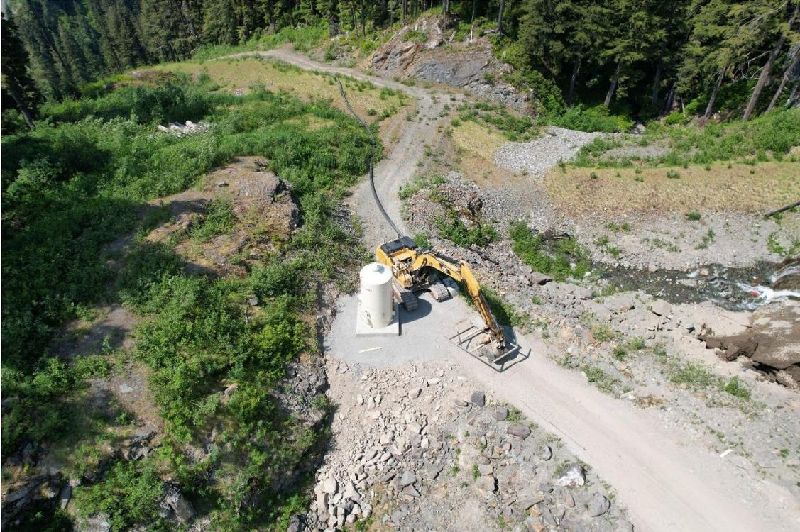
**Figure 5 – New water treatment plant clarifier foundation pedestals and lime silo foundations**
