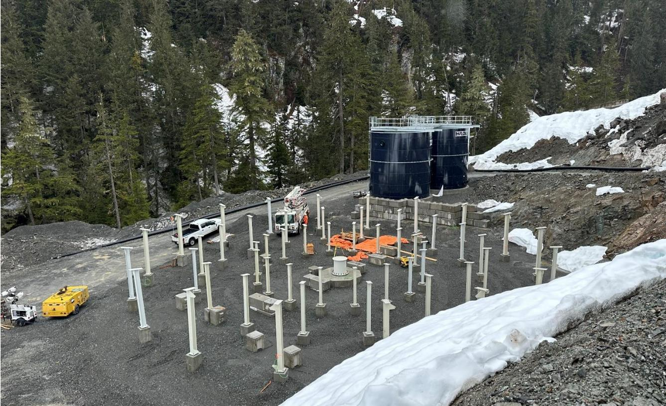
**Figure 7 – New WTP MBBR tanks installed**
