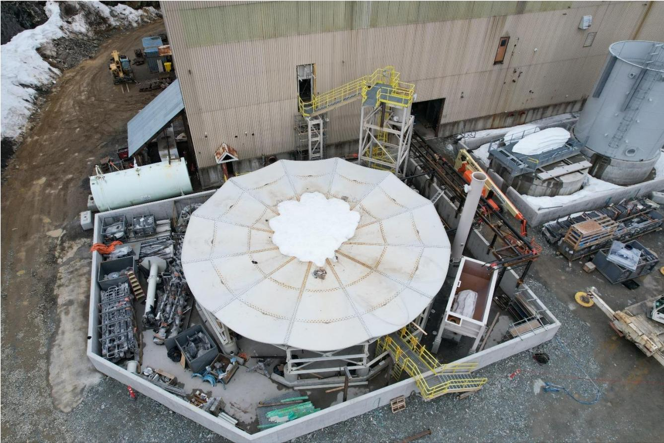
Figure 4 – Temporary WTP for tailings facility Spring water discharge
