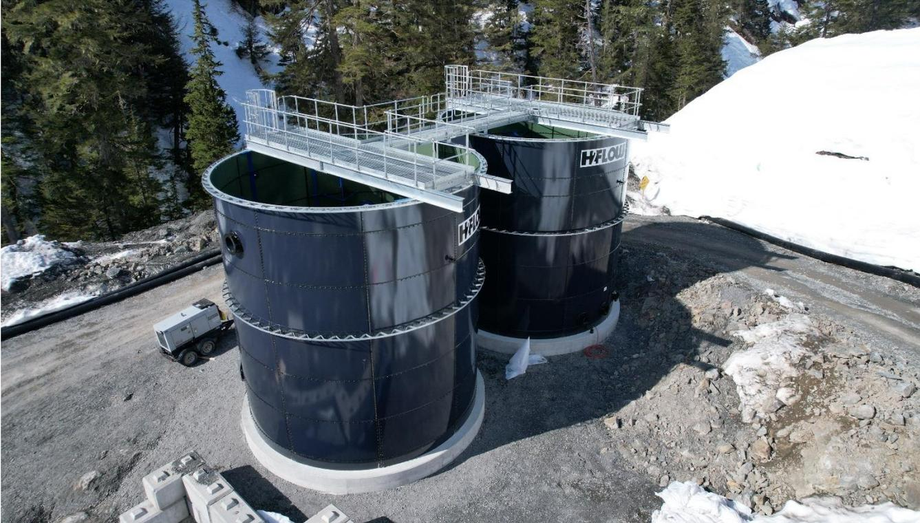
**Figure 6 – New WTP clarifier foundation pedestals installed**
