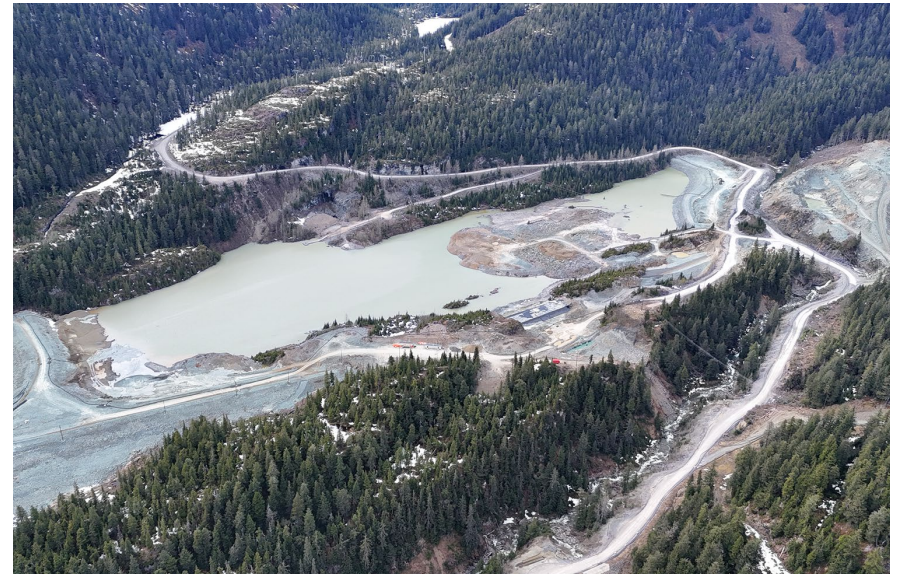
▲ TSF construction completed in early 2024
