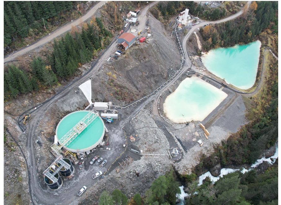
▲ New water treatment plant
