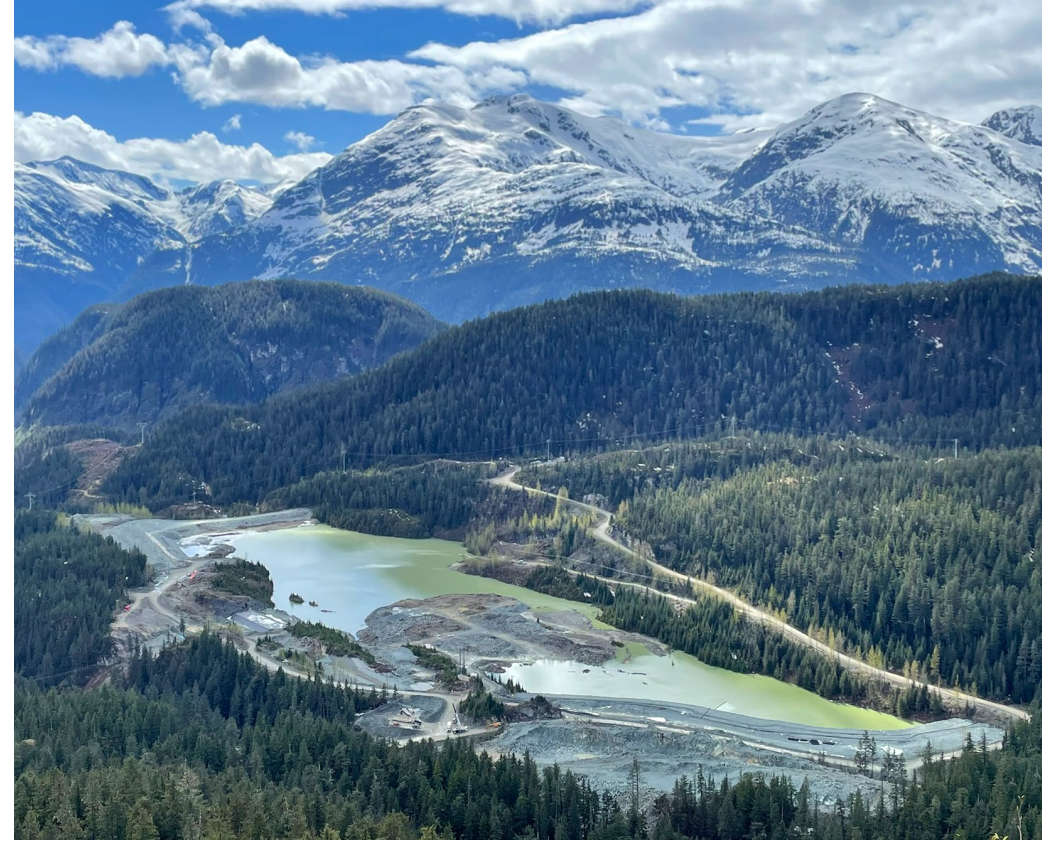
▲ Completed Tailings Storage Facility
