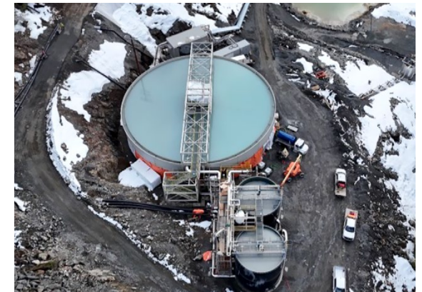
▲ Overhead views of the new Water Treatment Plant clarifier and lime silos ▼
