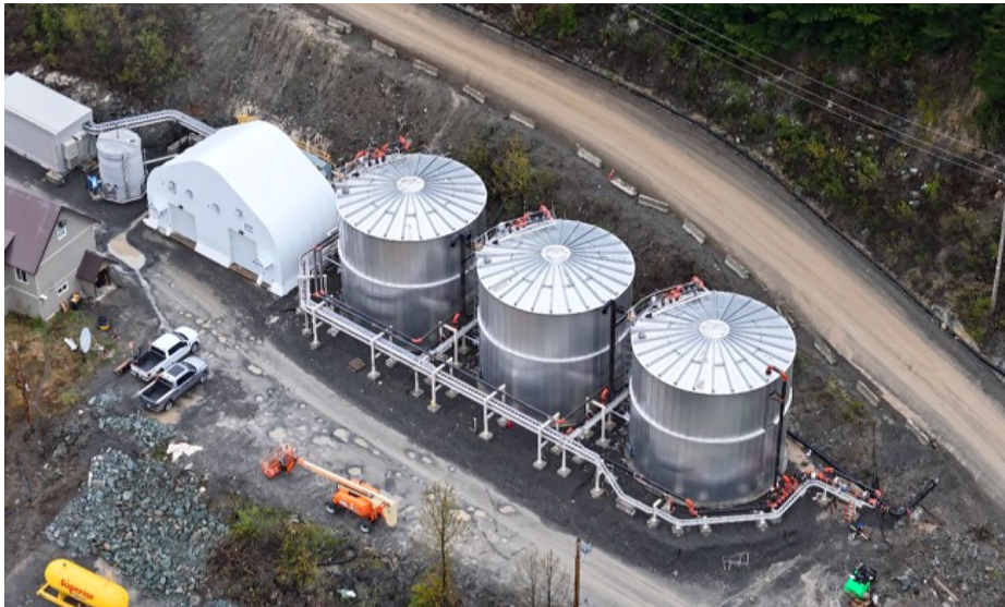
▲ Newly constructed Moving Bed BioReactor (MBBR) tanks
