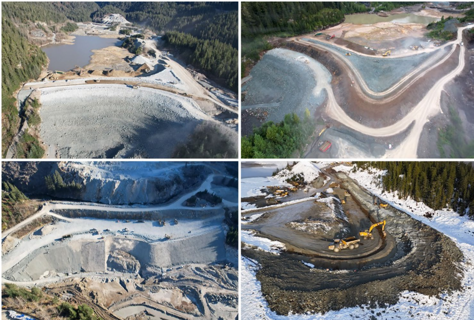
▲ Tailings Storage Facility Construction
