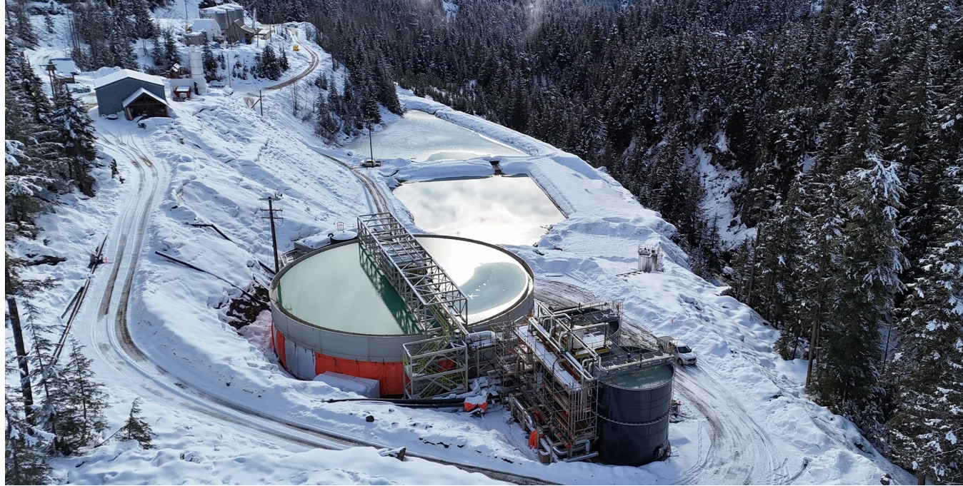
▲ Overhead views of the new Water Treatment Plant clarifier and lime silos ▼
