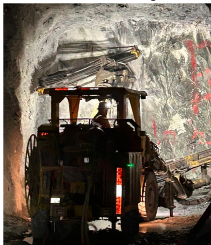
Figure 1. Underground development at the Premier Northern Lights mine
